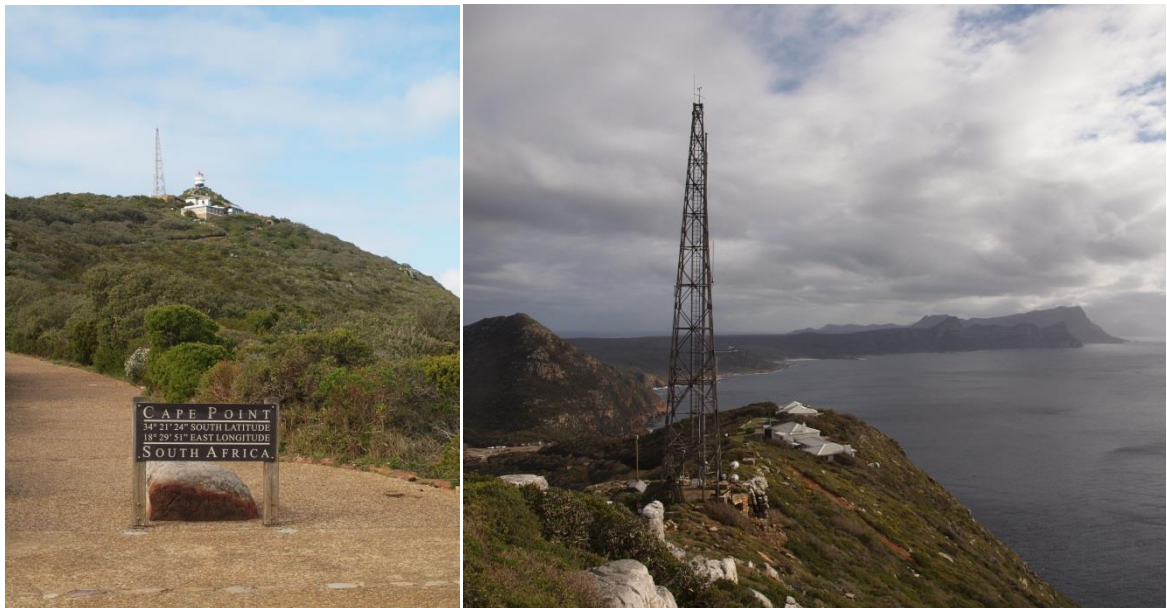
Figure 2. Views of the CPT building (left) and the 30 m tower (right) as seen from south to north.
